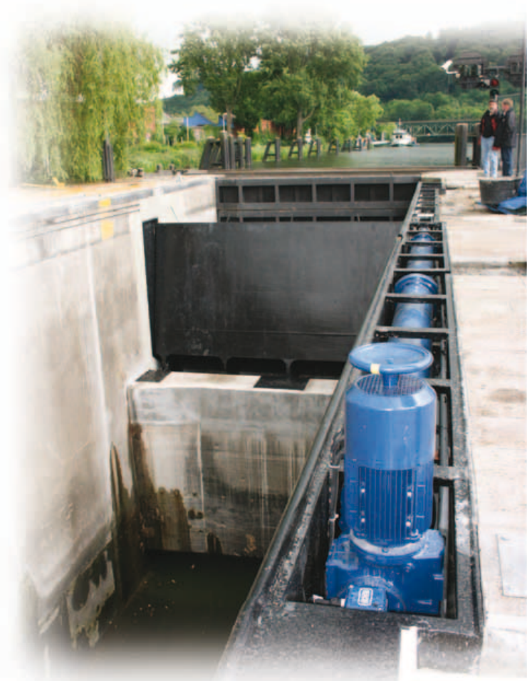
Segment gate operator, type: K1R9 SWB, Hub = 5.500 mm
