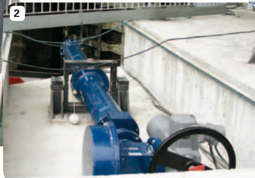
[1]-[3] Gate operator, type: K1R9 SWB with cardanic mounting option
