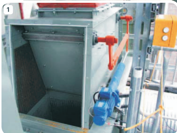
[1] Type T1A5 for a two-way chute in cement plant [2] Type T1K5 for a diverter gate in coal fired power plant
