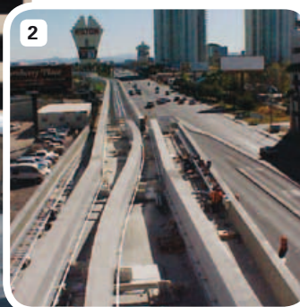
[1]-[3] Electric cylinders in the points of the monorail train in Las Vegas [4]-[5] Electric cylinders at the stop. Suspended monorail system, Dortmund university
