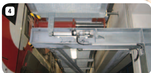
[1]-[4] Electric cylinders on service platforms
